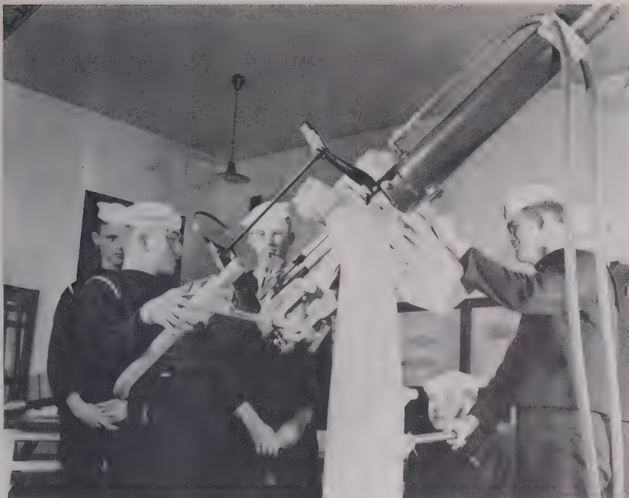
The 0.50-caliber water-cooled machine gun was the primary antiaircraft weapon of the interwar period. Here reservists train on one at the Washington, DC, armory, about 1940. Weapons of this type lined the gallery decks of US aircraft carriers early in World War Two; prewar they were mounted aloft in warships from destroyers to carriers.
