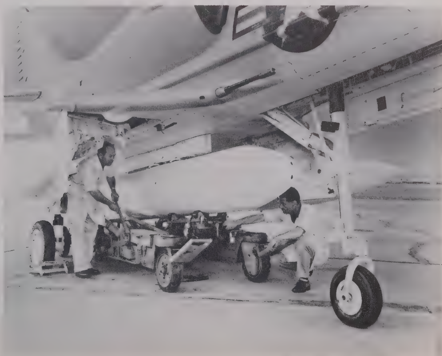
Postwar Navy air-to-air gun development was conventional, except for the introduction of the twin 20mm gun pod, shown here as it was introduced under an A4D-2 Skyhawk, with the conventional 20mm Mk 12 cannon evident in the wing root above it. The long tube above the wing is the aerial refueling pipe, leading to a nose probe.
