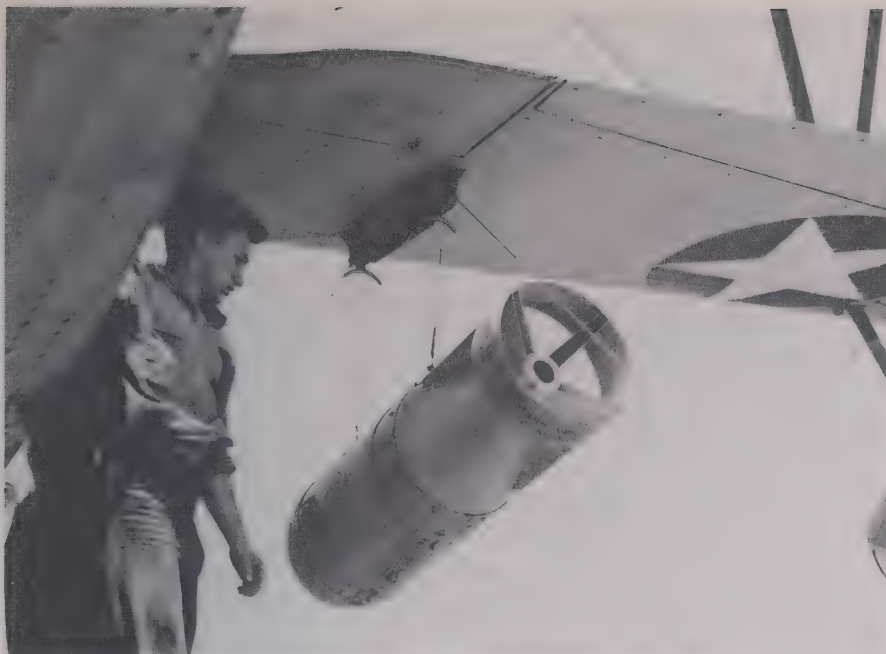
At first patrol aircraft carried adapted shipboard depth charges, but quite soon specialized aircraft types were evolved. This is a Mk 17 (325lb), the standard wartime aircraft depth bomb, being removed from a bomb rack aboard an SOC scout plane on the cruiser Philadelphia , 2 July 1942.
