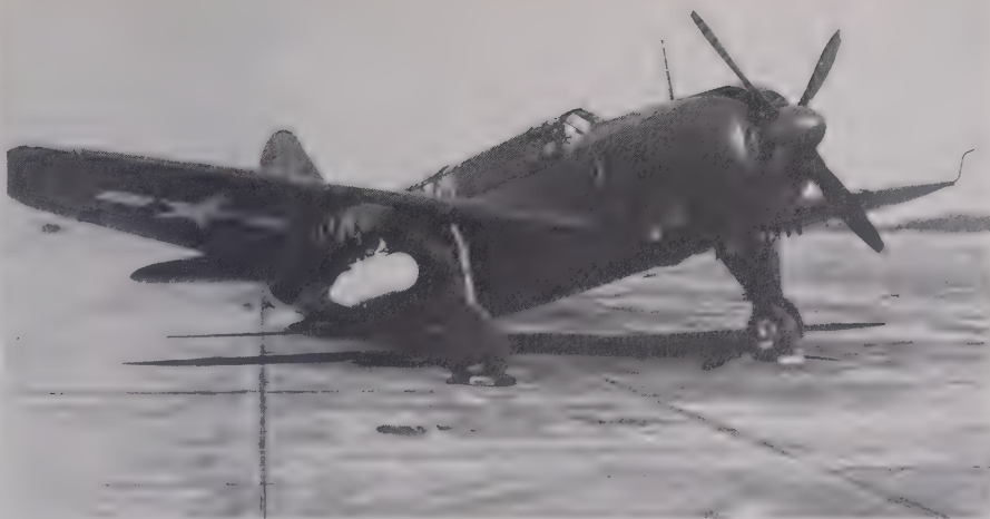
By 1945 all attack aircraft had internal fittings for APS-4 radar, which could be carried as an underwing, bomb-shaped pod. This is an SBF-4E, a Fairchild-built Helldiver, at Patuxent River, 17 December 1945. Similar pods were often carried postwar by Skyraiders. The zero-length rocket stubs outboard of the pod (and visible on the other wing) were also standard by this time.
