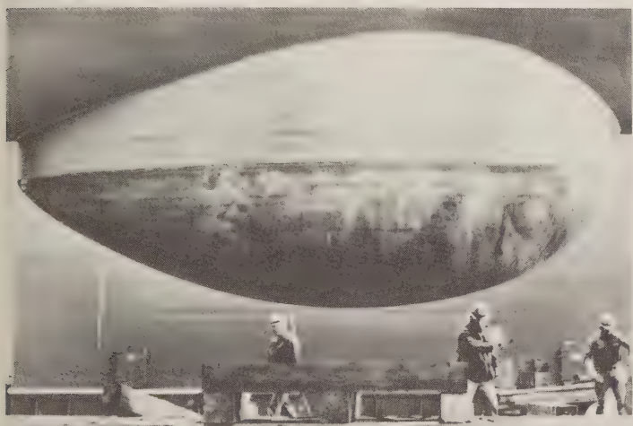
SQS-56 transducer and its sonar dome.
