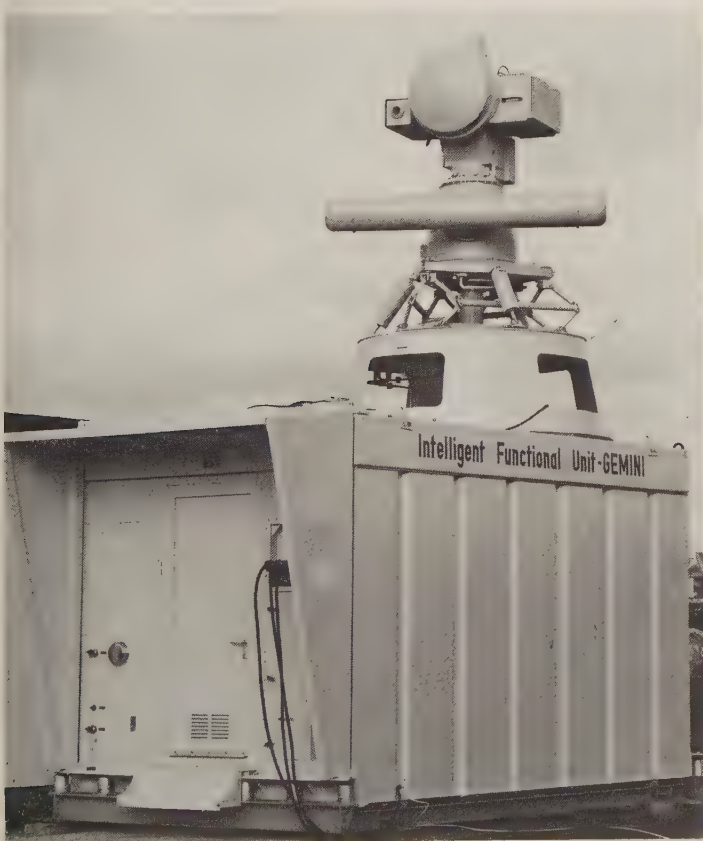
Gemini carries the X-band acquisition radar developed for Goalkeeper (the long slotted array) and a Ka-band tracker (as in LIROD) as well as a laser range-finder in 1990. The director can also carry a FLIR. Gemini has not yet been sold, but apparently it is now being marketed in container form. (Signaal)
