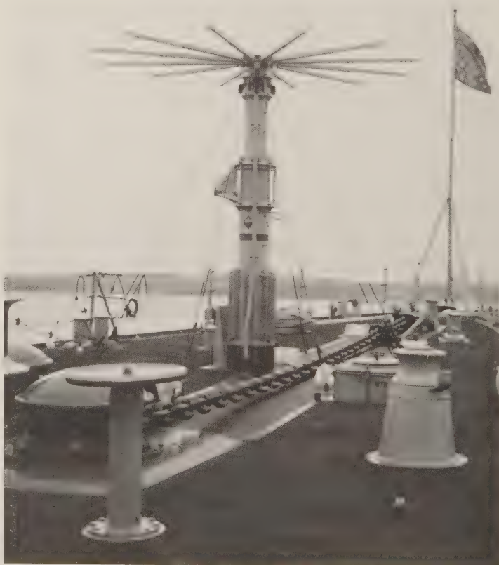
HF discone data-link antenna (AS-2865) for NTDS, USS Mississippi , June 1988. (Stefan Terzibaschitsch)
