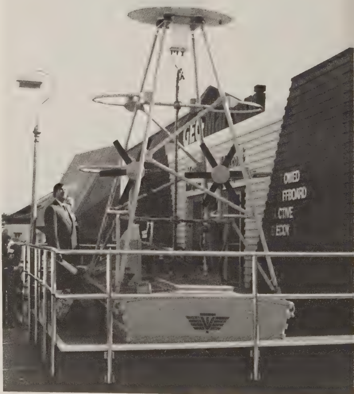
The Marconi towed decoy (TOAD), on display at RNEE 1989: the jammer in the radome is powered by the 2 propellers, which turn as the small boat carrying the decoy is towed through the water. The boat hull carries the Vosper-Thornycroft logo. (Author)
