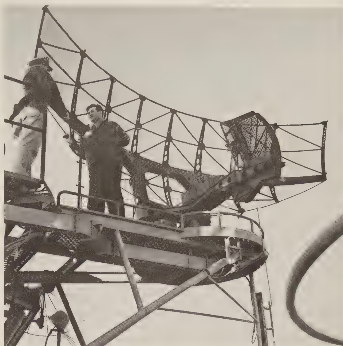
Although SPS-6 is virtually extinct in the U.S. Navy, many survive abroad. This photograph was taken in 1950, but current installations use the same antenna, typically at the masthead. (U.S. Navy)
