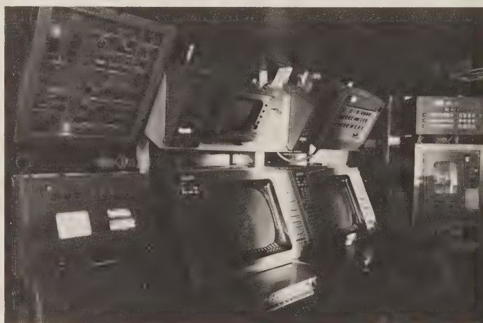
TAVITAC CIC, showing the command-and-control consoles in place. (Thomson-CSF)
