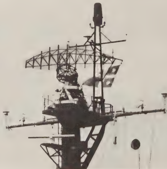
CWS-3 antenna. The minelayers have CWS-2, whose antenna resembles that of the Italian RAN-10S but is wider. (U.S. Naval Institute)
